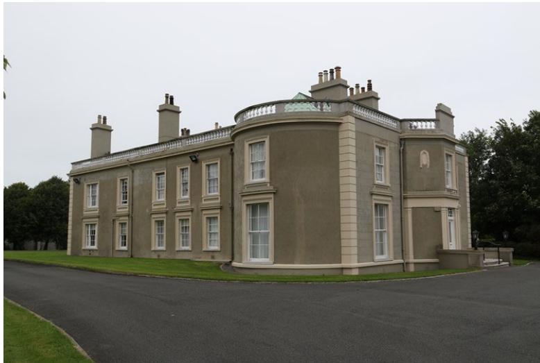
Plate 5: Sybil Hill House, with southern elevation at right and western elevation at left
