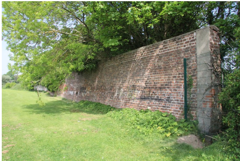
Plate 10: Brick-faced wall near northern boundary
